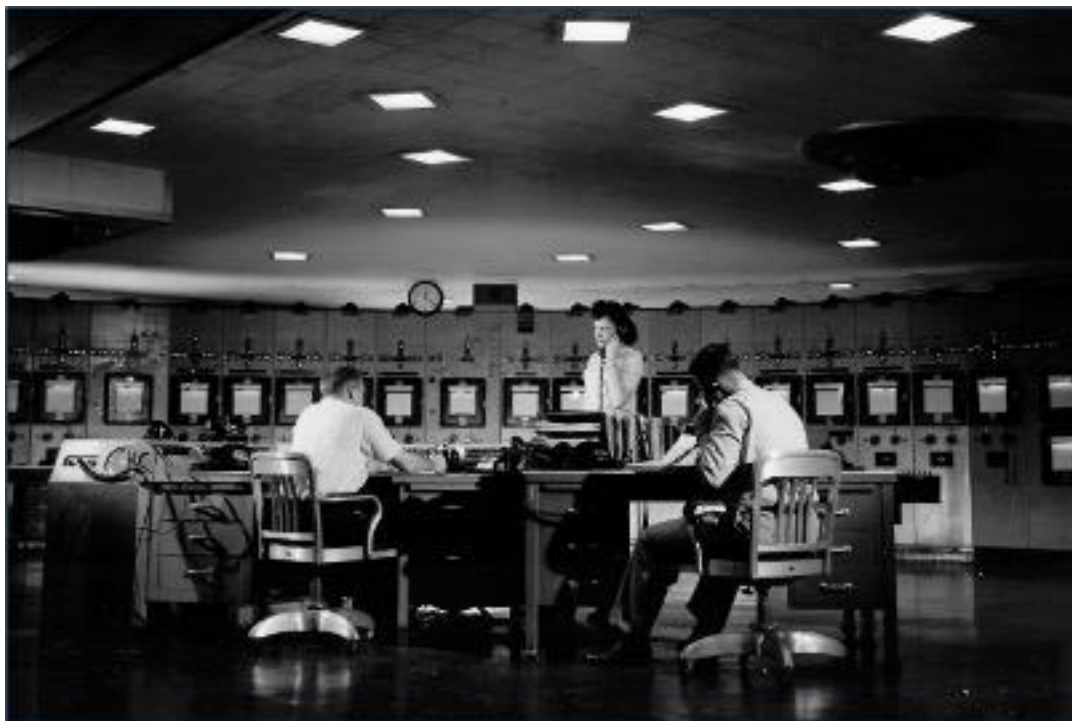
K-25 Gaseous Diffusion Plant, Clinton Engineer Works, Oak Ridge TN The Control Room was the most advanced, most fully instrumented plant of its time. (Public domain Courtesy of Barbara Scollin)
